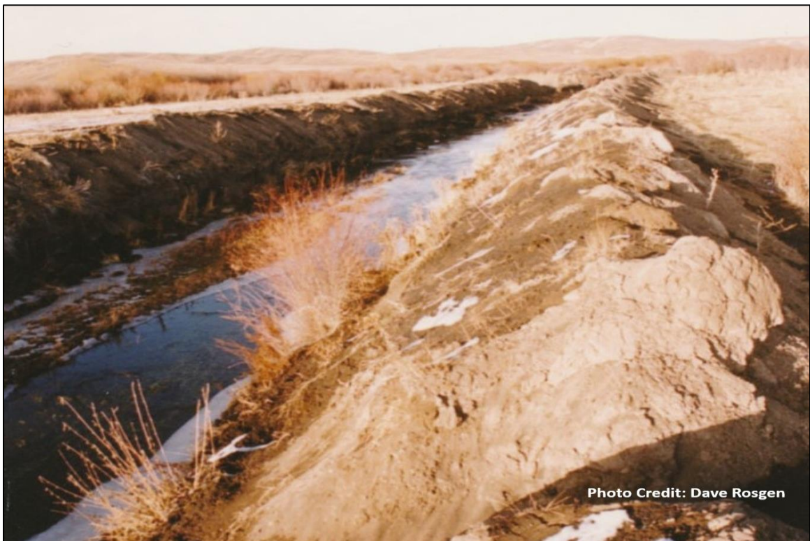
Photograph B20. Channel Straightening/Berm Construction
