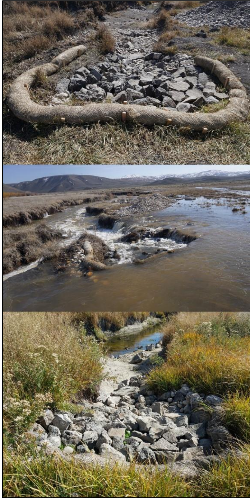
Photograph B24. 2022 Repair at Time of Construction, During 2023 Flooding, and Post-Flooding
