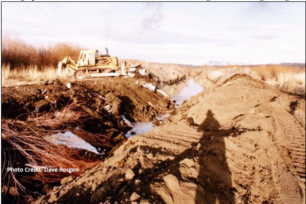
Photograph B22. Active, Plug and Pond Restoration of Straightened Channel Incision
